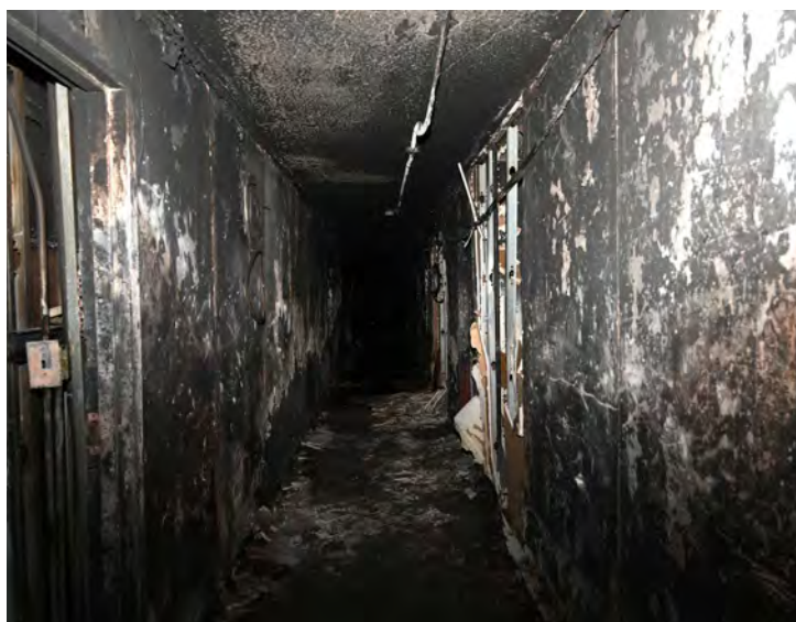
Public hallway of the third floor at Bronx Box 55-3162 on January 9, 2022. (Photo by the FDNY Bureau of Fire Investigation)
