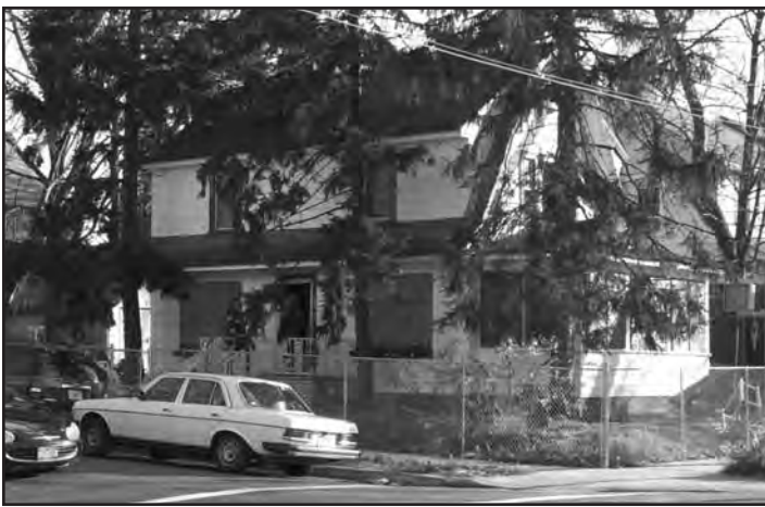
Photo #4--187-02 Newburg Street. Corner view of the private dwelling as units saw building. Heavy fire showed in side cellar window on exposure #2 side cellar windows.
