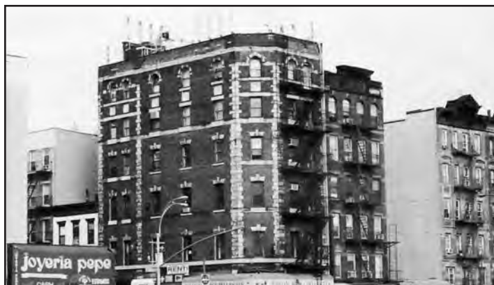
Antennae situated above the perimeter walls at the roof level are a visual indication of a cellular phone communication site.
